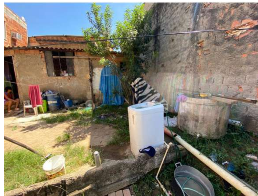
4. Front yard with open sewage and accumulated waste.
