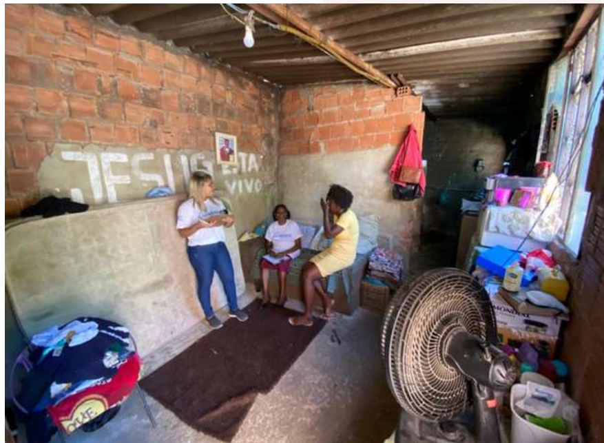
3. Precarious structure with exposed sewage and electrical hazards.
